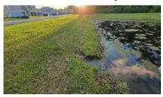
Action Item Description c3 - eroding valley in pond bank. recommend that washout be filled and sod added to repair.
