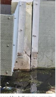
C3 - side skimmer panel has half missing. opposite end concrete corner is cracked. wide pond side skimmers may be loose.
